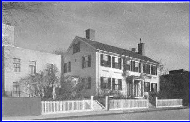
Figure 2 Cambridge School of Architecture and Landscape, Cambridge, Mass.; Torrey Hancock House (1827) at right, offices and drafting room wing by Eleanor Raymond et al., 1928 (brochure, Smith College Archives, Smith College)
