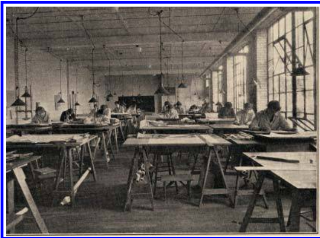
Figure 10 Cambridge School, drafting wing interior ( Cambridge School Bulletin 1, no. 1 [Dec. 1928], Smith College Archives)
