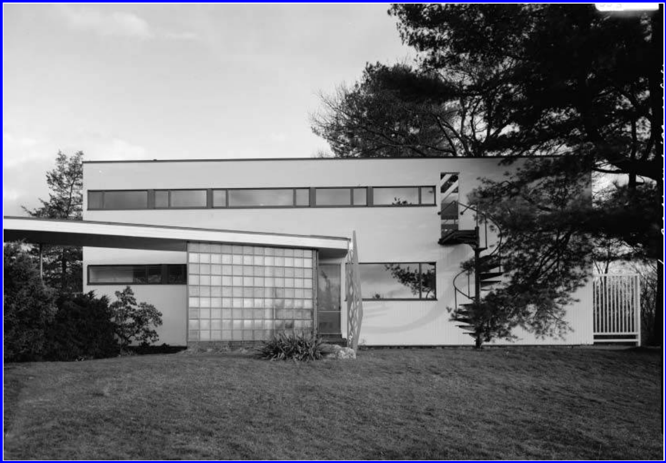
Figure 1 Walter Gropius, Gropius House, Lincoln, Mass., 1938, from north (photo: Jack Boucher 1986, Historic American Buildings Survey, HABS MA, 9-Lin 16-7, Library of Congress, Washington, D.C.)
